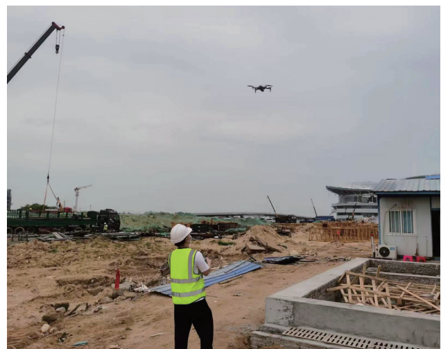
Using drones to inspect the construction site
