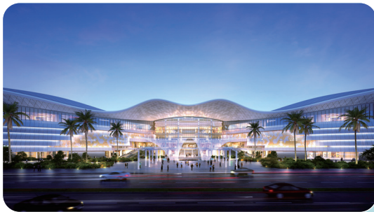
Haikou International Duty Free Shopping Complex (under construction)
